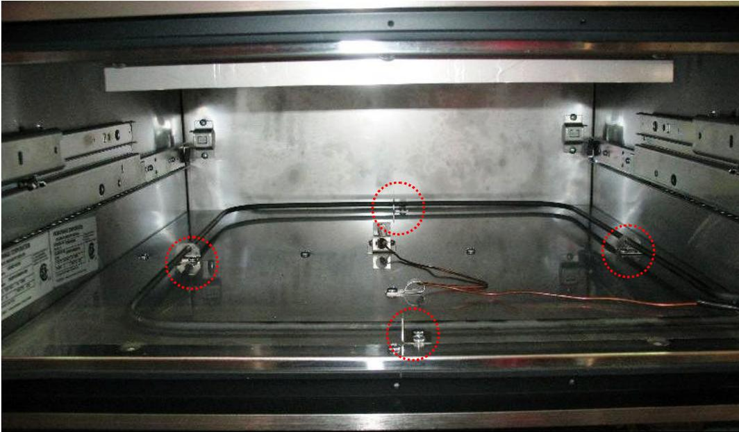
FIG 12 shows the right side entrance where the thermostat and heating element enter the chamber of the warming drawer. Remove the (2) screws shown to pull the heating element from the unit.
